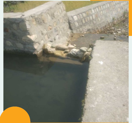
Outlet (Stone pitching)
